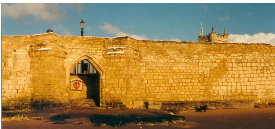
TOWN WALL GATE TO FISH SANDS
