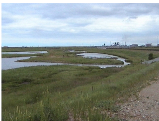
VIEW ALONG GREATHAM CREEK SEA WALL
