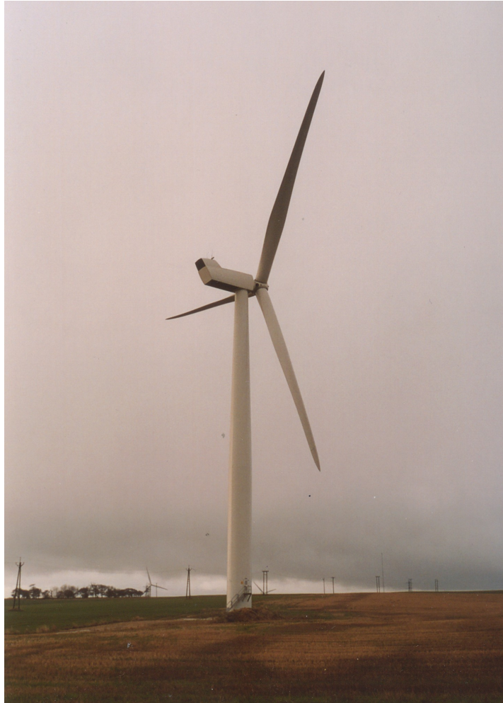
HIGH VOLTS WIND FARM, NEAR ELWICK
