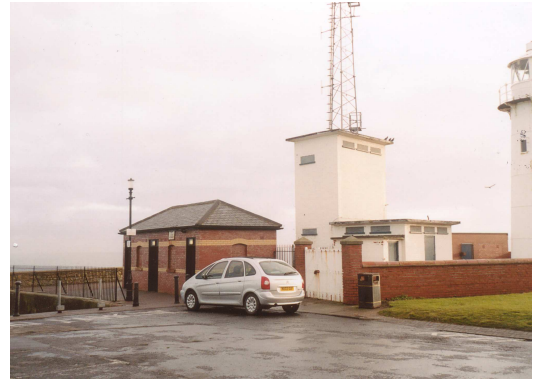
HEUGH LIGHTHOUSE, HARTLEPOOL HEADLAND: The proposed location for the new observatory building is on the seaward side of the disused Coastguard Lookout (centre), by kind agreement with PD Teesport.
