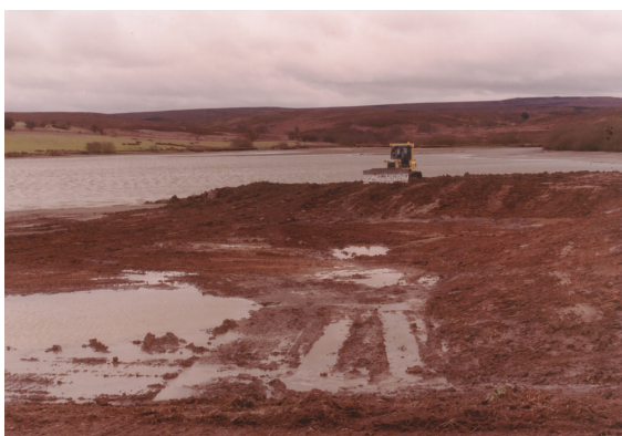
EXCAVATION OF THE SCRAPE
